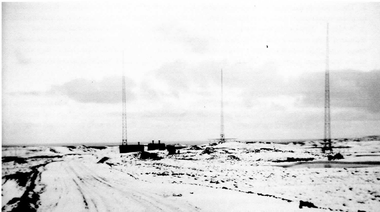
Radio range station and antenna towers. Building with two stacks contains Diesel generators
