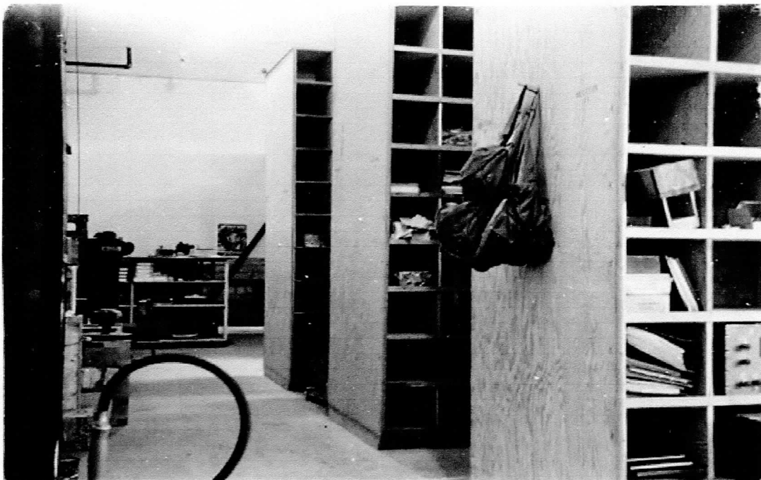
AACS 1946 Maintenance & Supply Room
