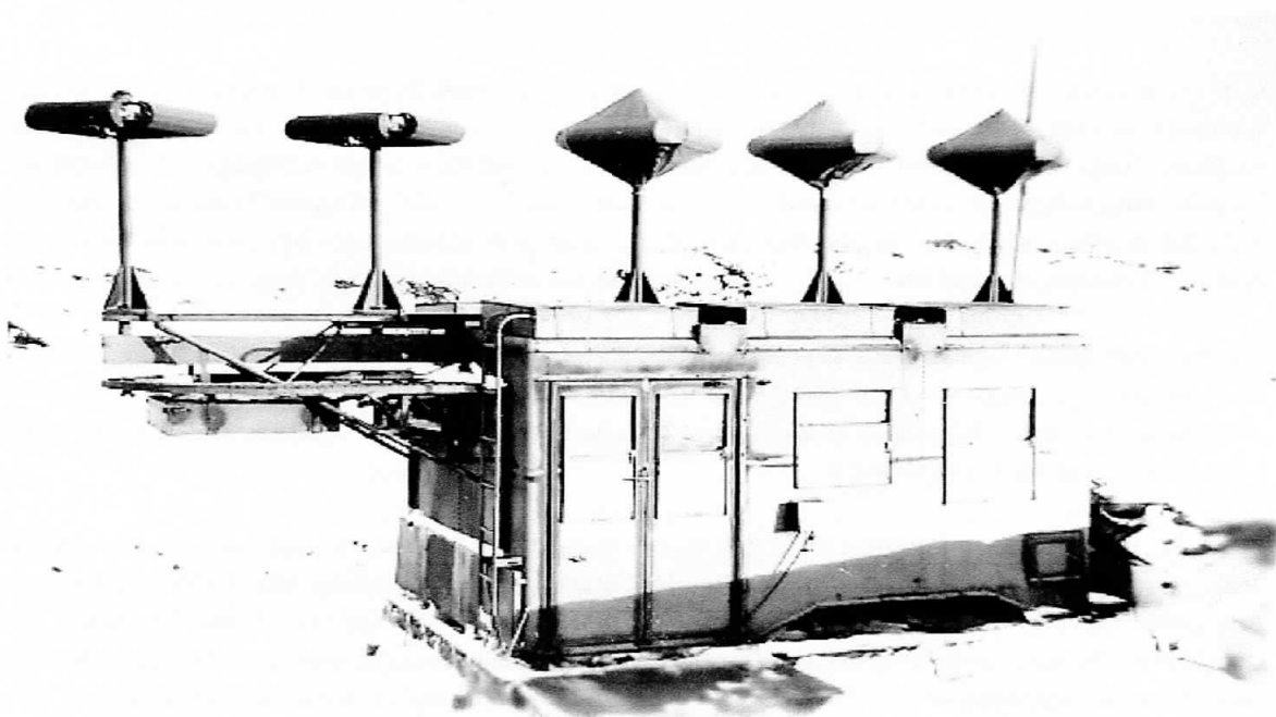
Moveable Localizer Transmitter with antennas on top
