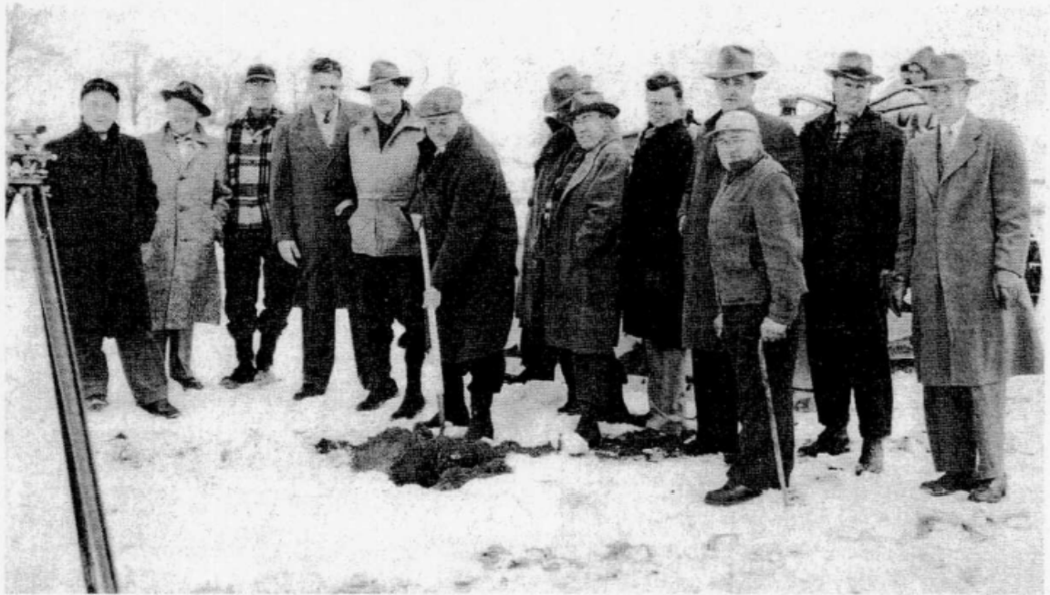
Everyone was smiles for the groundbreaking of Otsego Memorial Hospital's new building. Among those gathered were (l-r) Nick Strolle, C.O. Reed, Doug Enders, Mel Freel, Harley Nash, Boyd Baird, Jack Krause, Bob Audrain, Allen, and three unidentified persons.
