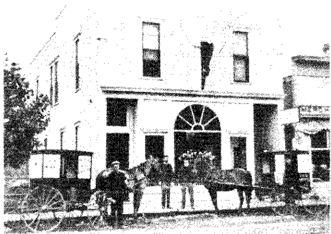
Post Office and Rural Delivery force on South Otsego Street.
