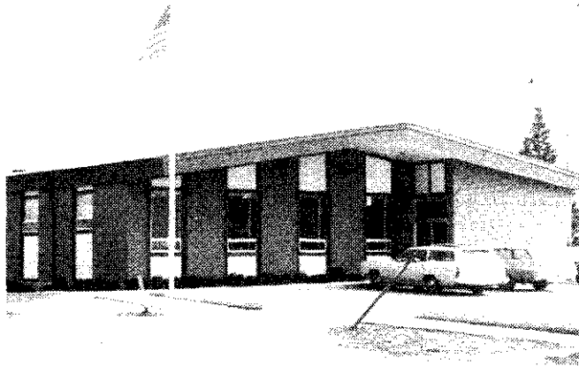
The United States Post Office in Gaylord is Sectional Center for all the 497 area and processes mail for 76 offices. A new addition to the present facility opened this Spring. Robert Fritz is Post Master.
