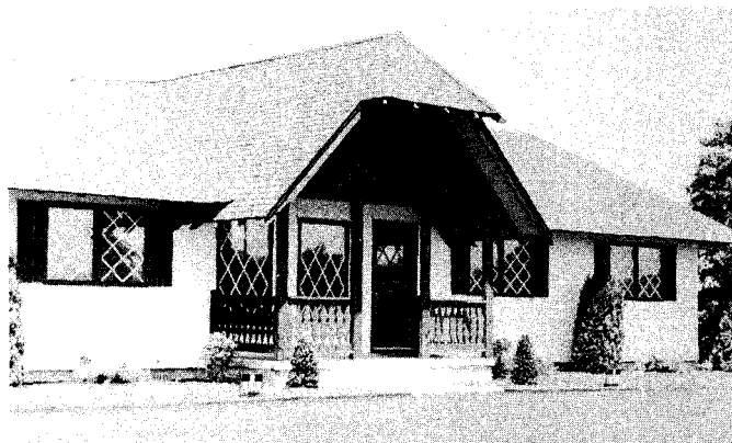
Shell Oil Office Gaylord M-32 East
