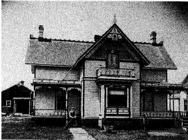
AROUND 1900 this is the way the Wells home looked at 212 South Otsego. In recent years it has been the home of the late Harry Lynch, and Mrs. Lynch. The curly-ques are now gone, but you will recognize the house when you drive by.
