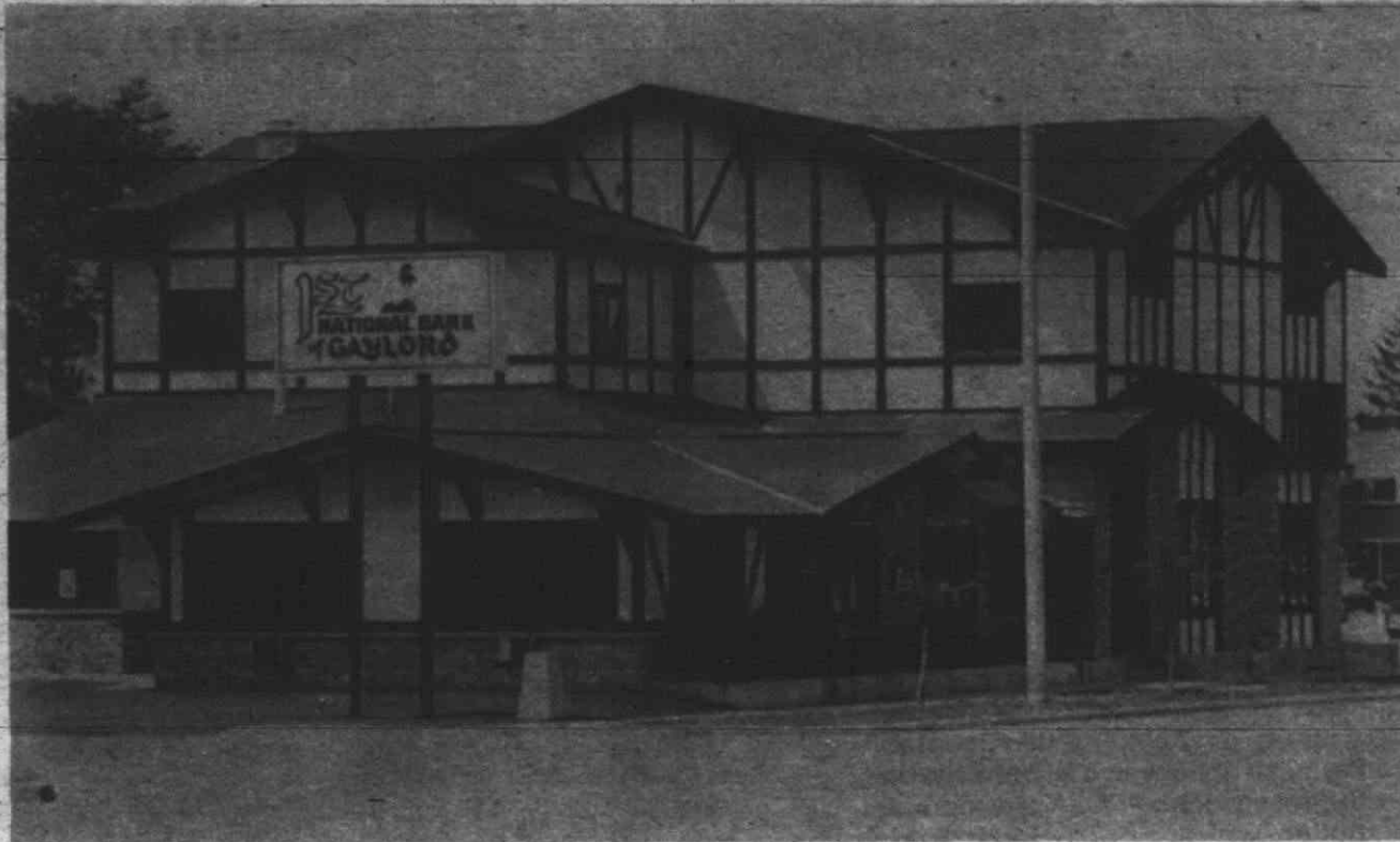
Main Office 501 West Main
